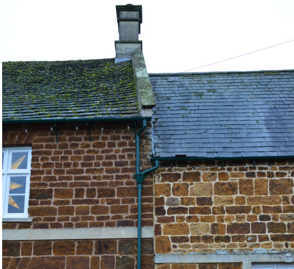
All Saints House - locally sourced stone building materials
