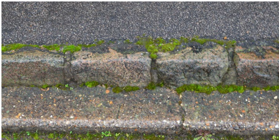
Granite Sett Kerb Stones
