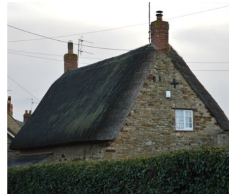
12 Church Street with traditional long straw thatch
